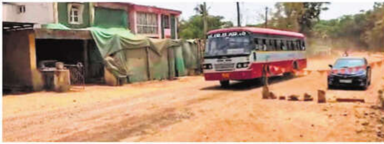
The pathetic condition of dust-emitting road between Sirsi and Hubballi | EXPRESS
