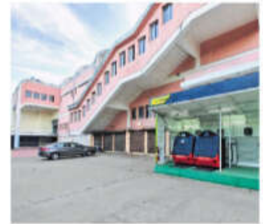
The swapping system lets drivers replace old ones instead of recharging | EXPRESS
