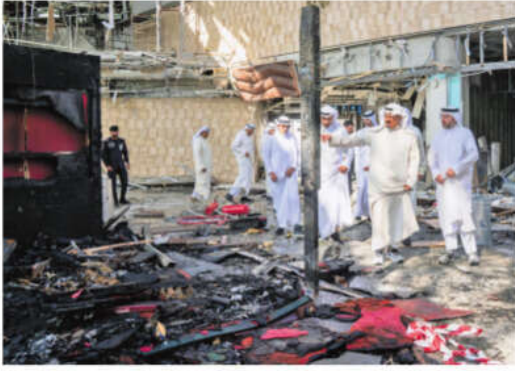
Kuwaiti Prime Minister Sheikh Ahmad al-Abdullah al-Sabah inspecting the damaged airport on Wednesday after an Iranian attack in Kuwait City | AFP
