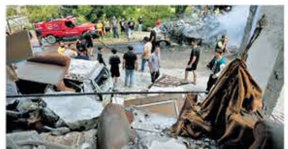
People inspect the damage following Israeli bombardment on a building in the village of Saksakiyeh in southern Lebanon | AFP
